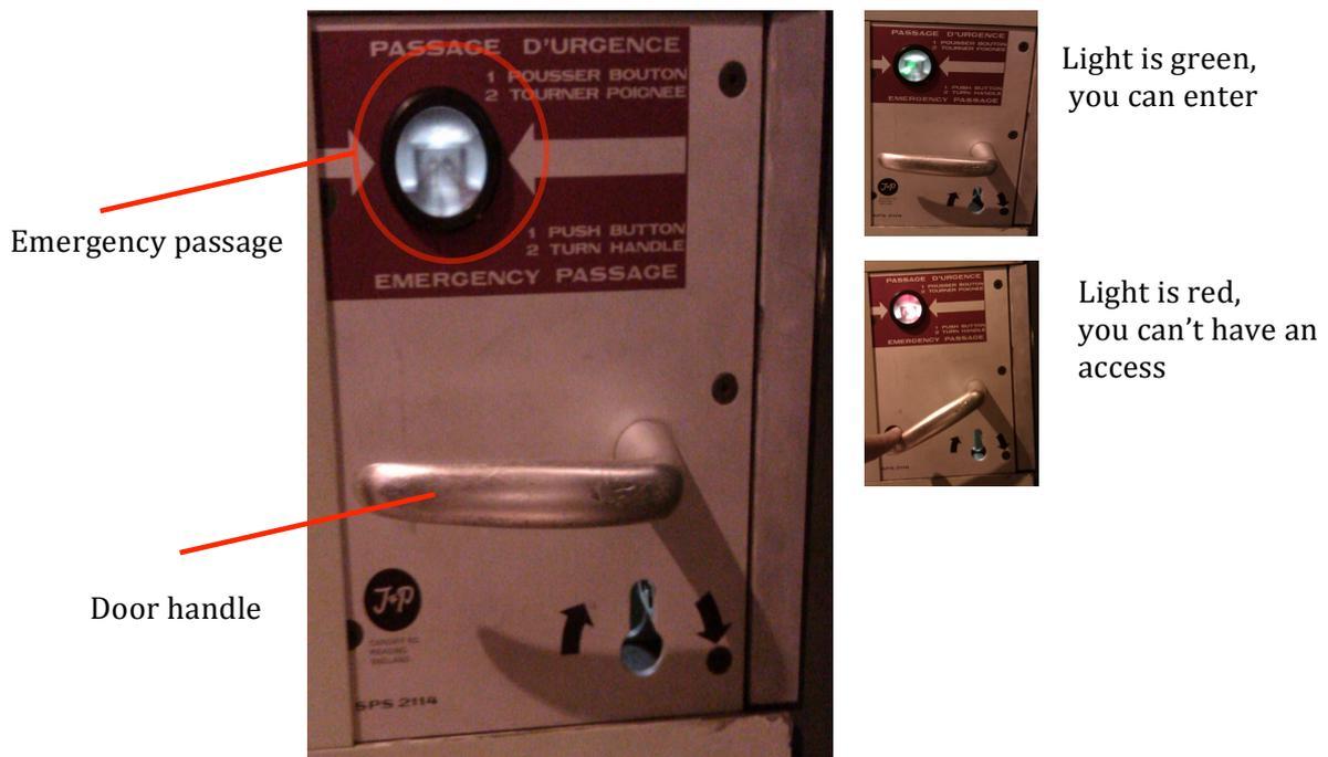
**Figure 2** — Detail of a PPE door lock.
